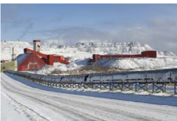
Coarse ore stockpile with #2 conveyor in foreground.
