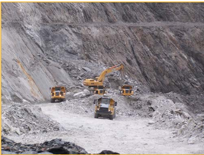
Carman Construction mucking Blast 22 in the Dome Pit.
