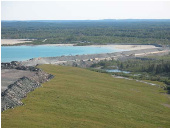
The above photo shows the north and west dams in the background and successful reclamation of one of the waste dumps in the foreground
