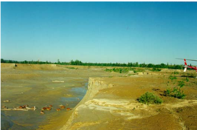
Phase I area of Coniaurum Tailings prior to rehabilitation
